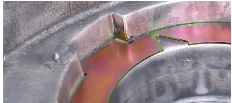
The protector in place, pump's load spread over large surface area
